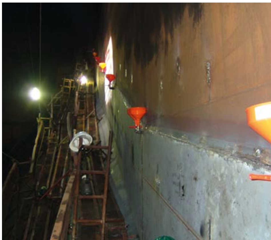
Crack repair and reinforcement
