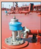
Fixed installed tank cleaning machines
