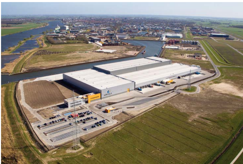
Wärtsilä has consolidated its European service warehouses at kampen, The Netherlands.
