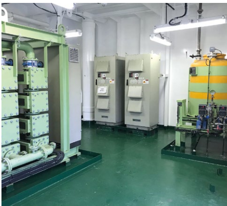
A Hyundai BWTS installed by ASRY on a VLCC
