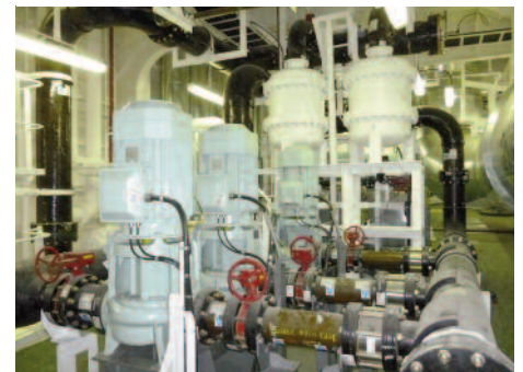
Wash water treatment plant, open-loop system. Source: EGCSA
