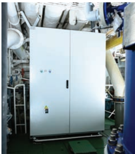
The control cabinet can be fitted up to 150 m away from the system.
