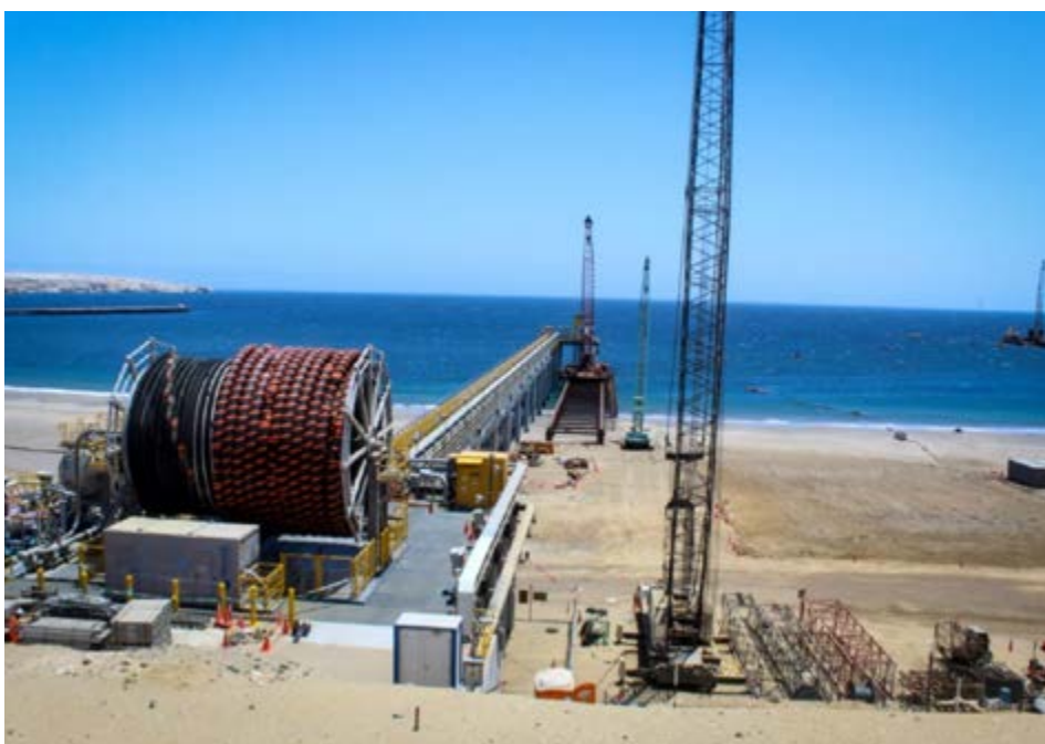
Chemiline being used for ship to shore transfers of sulphuric acid in Marcona, Peru
